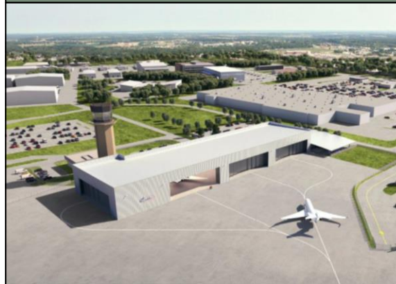
Republic Airport | Farmingdale, NY 400k SF hangar development
