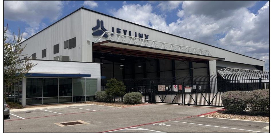
San Antonio Airport | San Antonio, TX 7-hangar, 126k SF hangar facility
